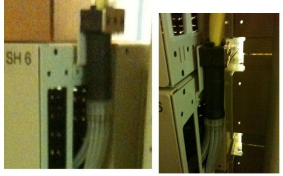
The transition piece has a label showing which side to face toward the panel.
