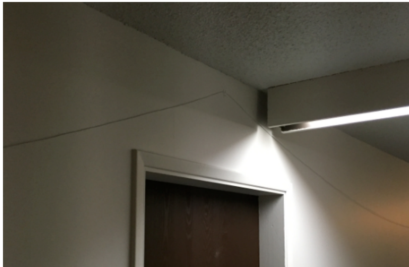
InvisiLight Multifiber Cord supported by a clip above a doorway before it is adhered to the wall
