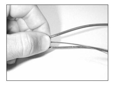
Figure 3 – Separate the fibers from the split buffer tube.
