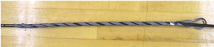
Figure 14 – Completed installation of the dead-end.
