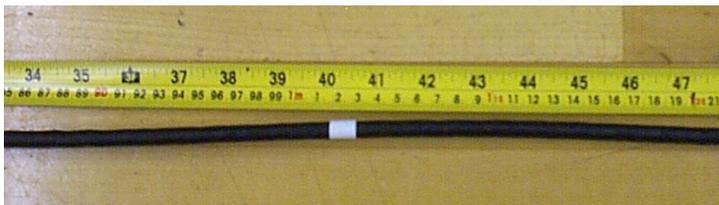
Figure 15 – Mark the length of cable jacket to be removed.
