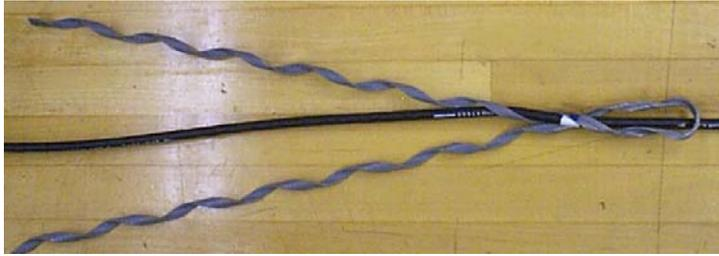
Figure 12 – Wrap the dead-end onto the cable.
