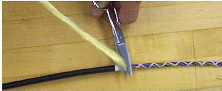
Figure 20 – Cut the strength members to length as required.
