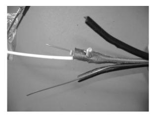
Figure 13 - Install bottom half of bond clamp.
