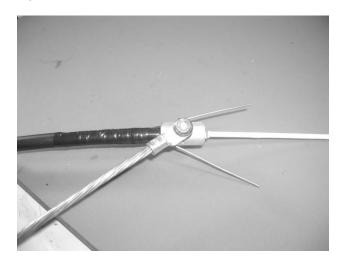
Figure 16 – Connect the bond wire to the bonding clamp.
