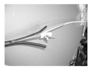
Figure 14 - Install top half of bond clamp.
