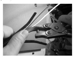
Figure 12 – Punch a hole in the armor.
