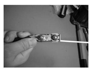
Figure 5 - Trim the strength wires and secure between the lock cap and extension bracket.
