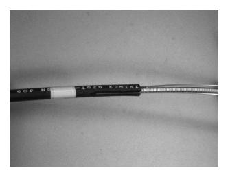
Figure 1 – Remove the cable jacket to expose the strength members and corrugated armor.
