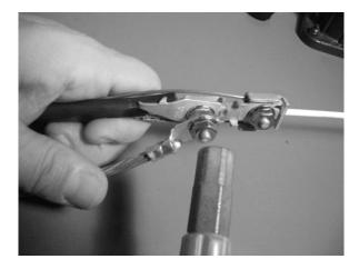
Figure 6 - Attach a bond wire to the bond clamp.
