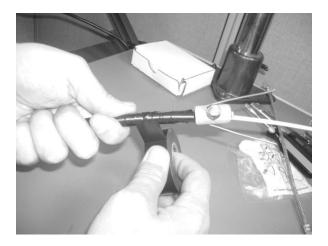
Figure 15 – Wrap the exposed strength members with vinyl tape.
