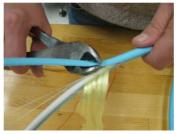
Figure 5 – Remove the outer jacket.
