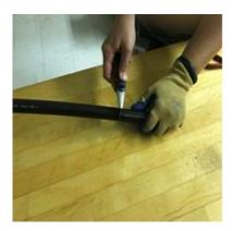
**3.4** Make two parallel slits in the jacket between the cable end and the adjacent ring cut. The slits should be approximately 180° apart. Remove the 4 inch section of cable sheath to expose the rip cords.
