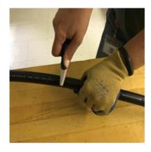
**3.3** Ring cut the cable a second time about 4 inches from the cable end.
