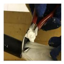
**4.6** Refer to the closure instructions to determine the length of core tube that is required inside the closure. Mark the core tube at the required length and use the 1050E core tube entry tool to slit the tube between the marks. Next, ring cut core tube at the marks and remove. Refer to OFS IP-054, *1050 Series Core Tube Entry Tools*, for further information on the 1050-type tools.
