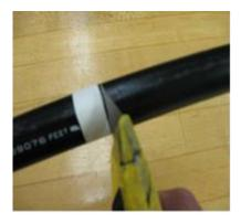
**4.2** At the center point of the section being opened, make two more ring cuts about 6 inches apart. Make two parallel slits in the jacket between the two adjacent ring cuts. The slits should be approximately 180° apart. Remove the 6-inch length of cable jacket between the adjacent ring cuts. Cut the rip cords in the center of the sheath opening.
