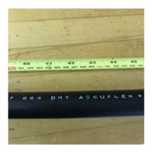
**3.2** Ring cut the cable at recommended stripping length.
