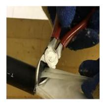
**3.8** Ring cut the core tube at the recommended length using a 1050E core tube entry tool. Refer to OFS IP-054, *1050 Series Core Tube Entry Tools*, for further information on the 1050-type tools. Remove the core tube to expose the ribbons and water blocking tape.
