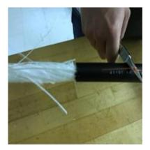
**4.4** While holding the strength members (rods and rovings) against the core tube, pull the cable jacket to remove.
