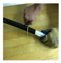
**3.6** While holding the strength members (rods and rovings) against the core tube, pull the cable jacket to remove.
