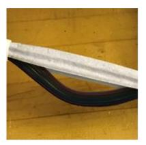
**3.9** Cut and remove water blocking tape to expose the fiber ribbons. Proceed as required with the closure assembly and splicing operations.
