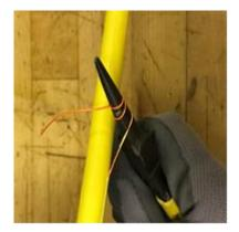
**3.7** Hold the strength members together with the core tube and pull the outer jacket to remove it from the cable.
