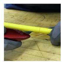
**3.5** Remove the 4-inch section of cable sheath to expose the rip cord.
