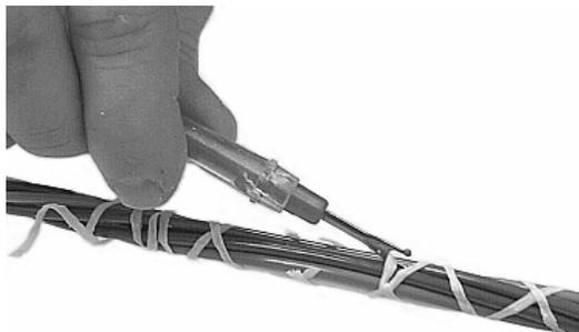
**Figure 35 - Remove the binder threads and water blocking tape.**
