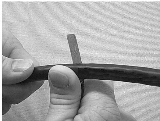
**Figure 2 - Ring cut the cable sheath.**
