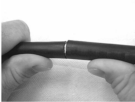
**Figure 3 - Separate the cable sheath.**
