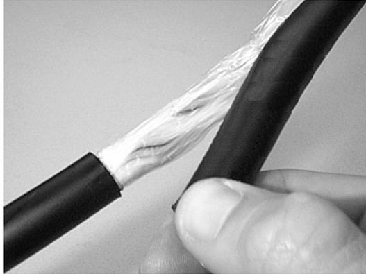
**Figure 27 – Remove the cable sheath.**
