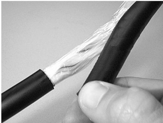
**Figure 8 - Remove the outer cable jacket.**
