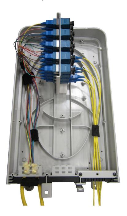
Fig.2 Typical installation of the "Fan-out" assembly
