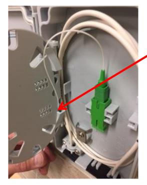
Pigtail placement on the bottom rear of the flip tray and is then routed counter clockwise on the front of tray. Pigtail length can be cut dependent on access to the fusion splicing equipment
