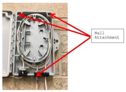
2. Attach the Indoor/Outdoor cable to the wall with EZ Cable Clip Shark Tooth Anchors. Place one of the anchors close to the enclosure to provide strain relief.
