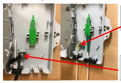
Strength Member Attachment with cable aramid yarn tied to grip the Indoor/Outdoor cable
