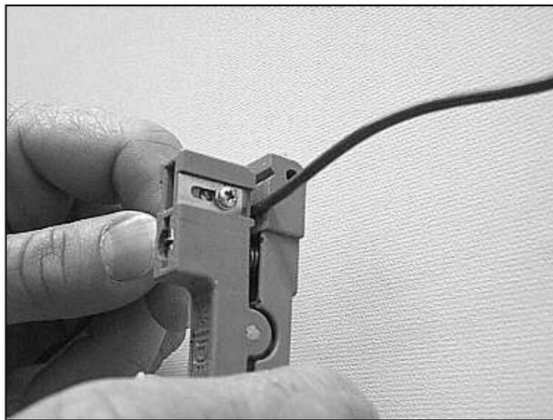
Figure 11A – Score the buffer tube with a buffer tube cutter.
