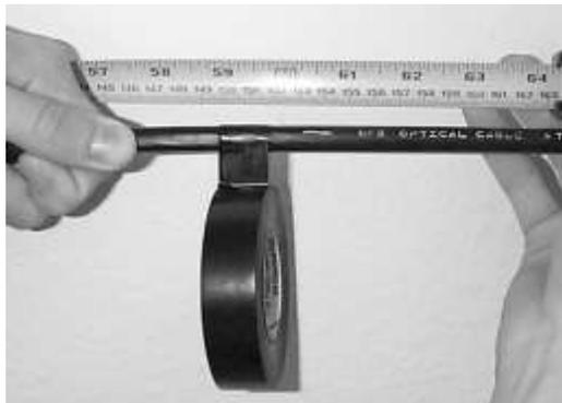
Figure 1 - Measure and mark the cable.
