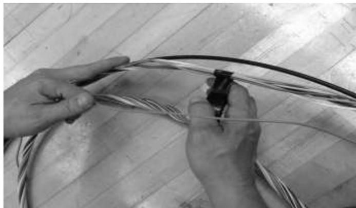
Figure 37 – Wrap a length of vinyl tape around the tubes at the ROL location.
