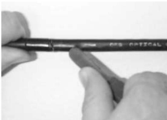
Figure 4 - Make a 5-inch longitudinal cut at the end of the cable.
