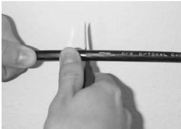
Figure 14 – Ring cut the cable jacket.
