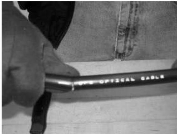
**Figure 23 – Flex the cable at the score marks to separate the sheath.**
