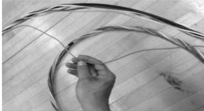
**Figure 48 – Unwind the buffer tube(s) that will be routed to the splice tray.**
