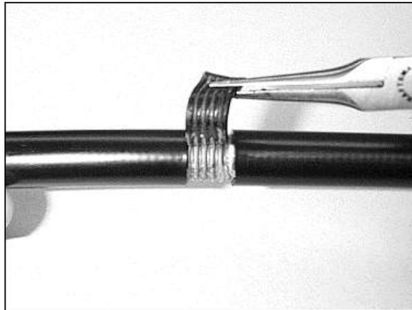
**Figure 25 – Remove the ½-inch section of outer jacket.**
