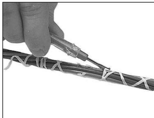
**Figure 39 – Cut and remove the binder threads.**
