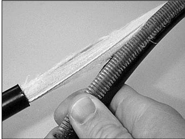
**Figure 7 – Remove the outer sheath and armor layer.**
