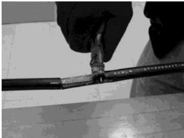
**Figure 5 - Remove the outer sheath from the armor.**
