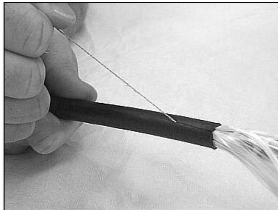
**Figure 36 – Pull the ripcord through the inner jacket.**
