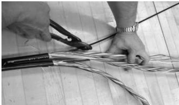
**Figure 53 – Cut the central strength member to length as required for clamping in the closure.**
