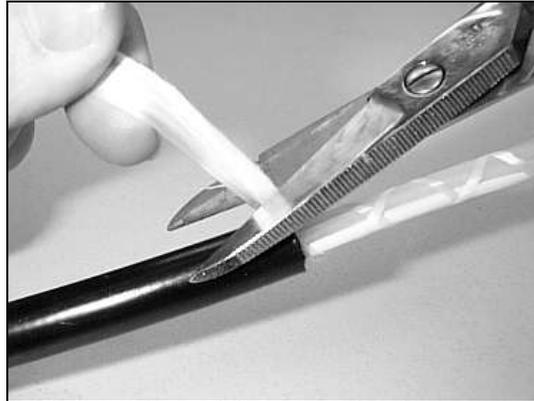
**Figure 37 – Cut and remove the dielectric strength members and water blocking tape.**
