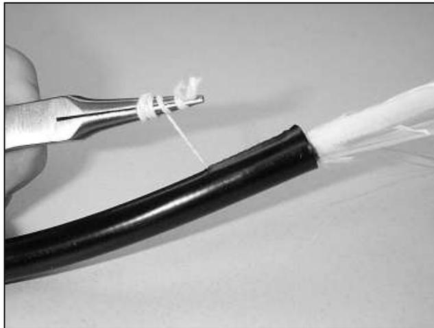
**Figure 8 – Pull the ripcord through the jacket.**
