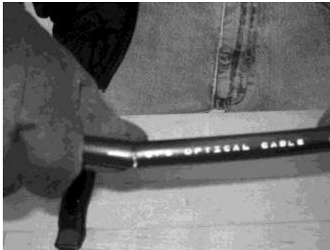
**Figure 3 - Separate the cable sheath at the ring cut.**
