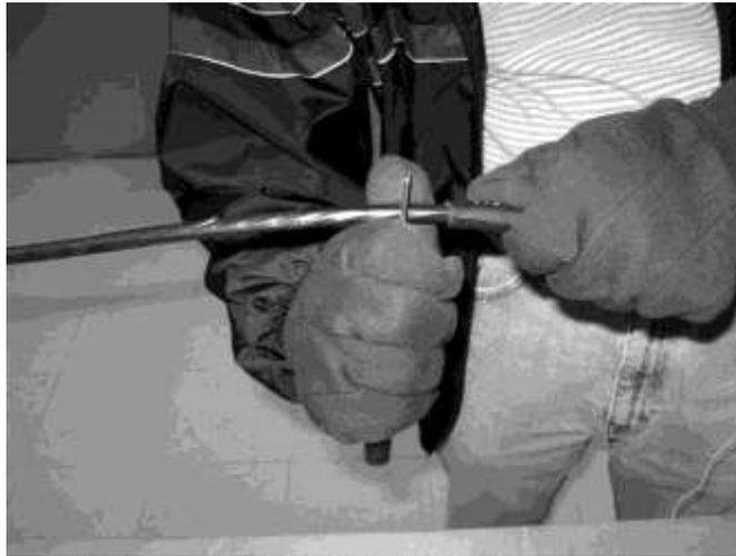
**Figure 11 - Ring cut the inner sheath.**
