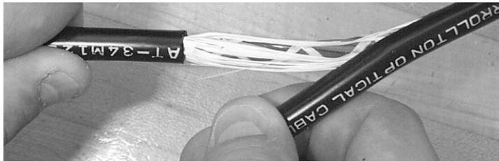
**Figure 7 - Remove the outer jacket.**
