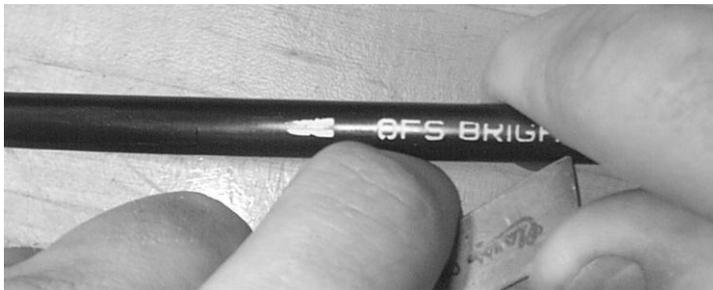
**Figure 19- Make a longitudinal cut between the two ring cuts.**
