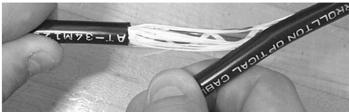
**Figure 20 – Remove the 10-inch section of outer jacket.**
