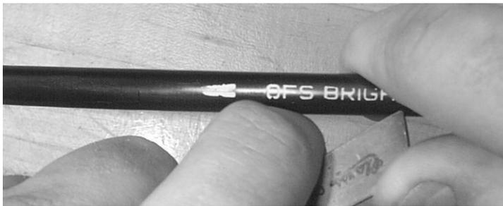
**Figure 4 – If necessary, cut the cable jacket longitudinally before removal.**
