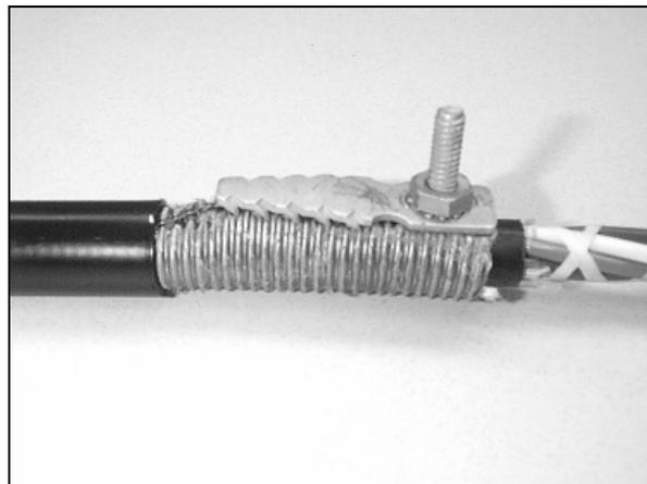
**Figure 16 - Install top half of bond clamp.**
