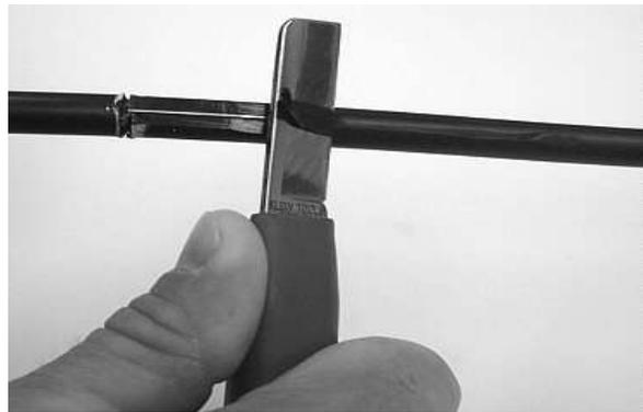
**Figure 3 – Shave the cable jacket to expose the strength members.**
