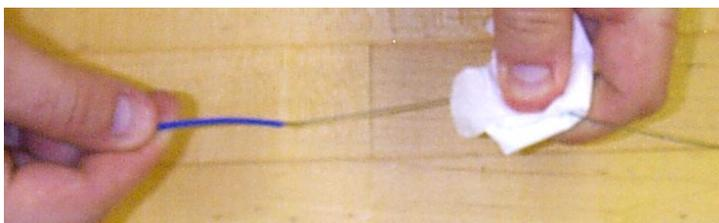
Figure 26 – Clean the optical fibers.
