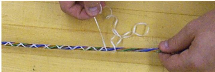
Figure 21 – Unwrap the binder threads from the buffer tubes.
