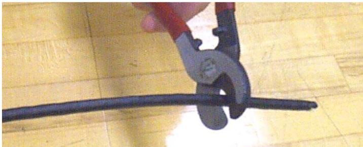
Figure 1 – Trim the cable end before attaching the grip.
