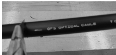
Figure 7 – Ring cut the outer jacket at both tape marks.
