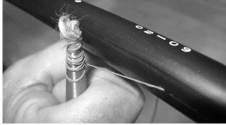
Figure 9 – Pull the ripcords to the opposite ring cut.
