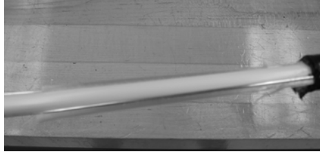
Figure 6 – Cut the strength members and copper wires as required.
