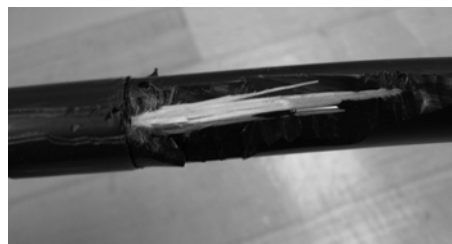
Figure 8 – Shave the outer jacket to expose the strength members and ripcords.
