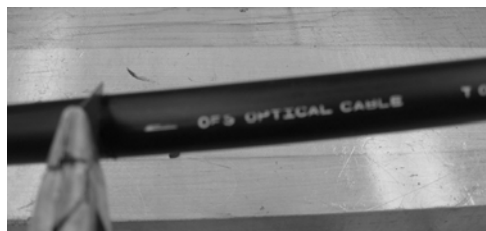
Figure 1 – Ring cut the outer cable jacket.
