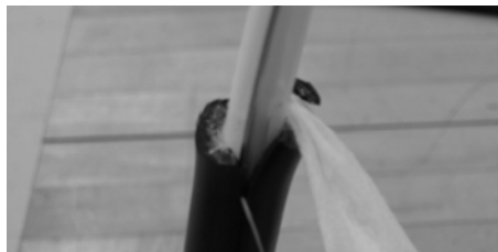
Figure 5 – Cut the rip cords and water blocking tape.
