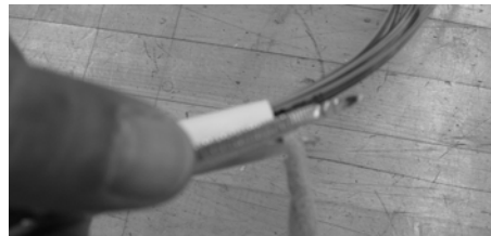
Figure 14 – Cut and remove the water blocking tape.
