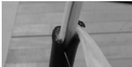
Figure 11 – Cut the rip cords and water blocking tape.
