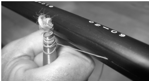
Figure 3 – Pull the ripcords through the outer jacket.
