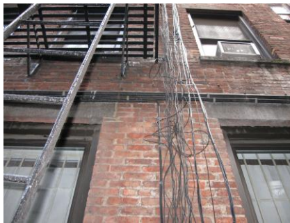
Confirm Bundled Cable Location.
