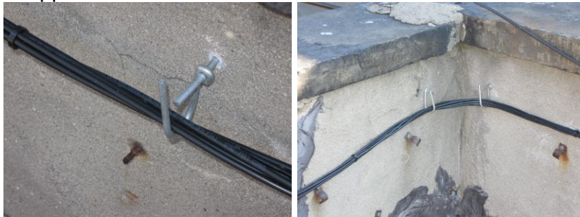
D rings for horizontal support on knee wall.
