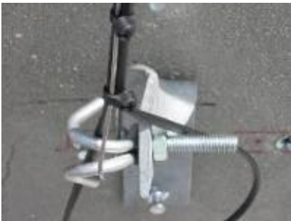
B Drop Wire Hook (Ram's Horn): 400315156
