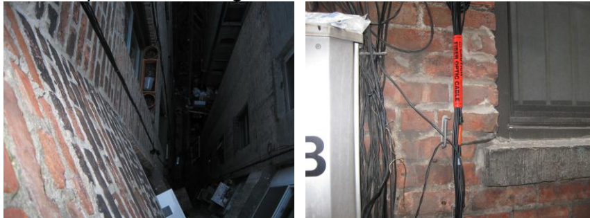
Orange alignment marker viewed from top of building and bottom window.
