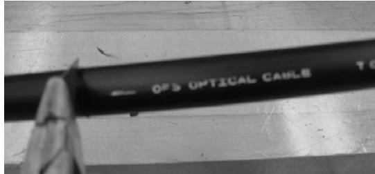
Figure 3 – Ring cut the outer cable jacket.
