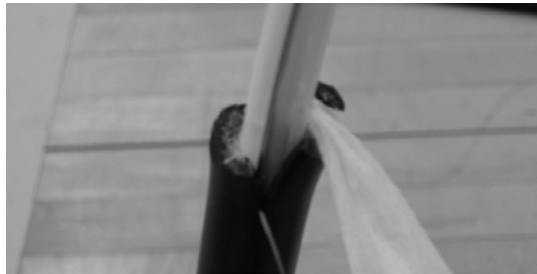
Figure 7 – Cut the rip cords and water blocking tape.
