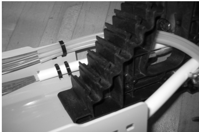
Figure 14 – Fasten transport tubes to storage basket.
