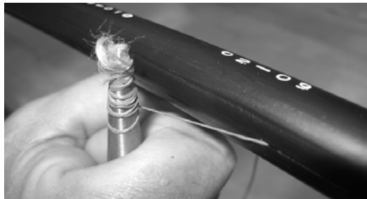
Figure 5 – Pull the ripcords through the outer jacket.
