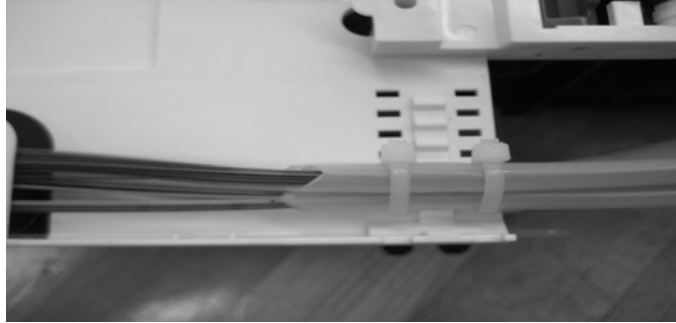
Figure 16 – Fasten transport tubes to splice tray.
