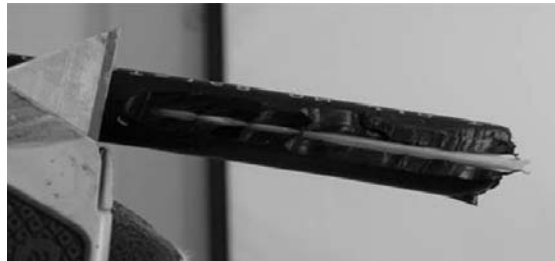
Figure 4 – Expose the strength members and rip cords.
