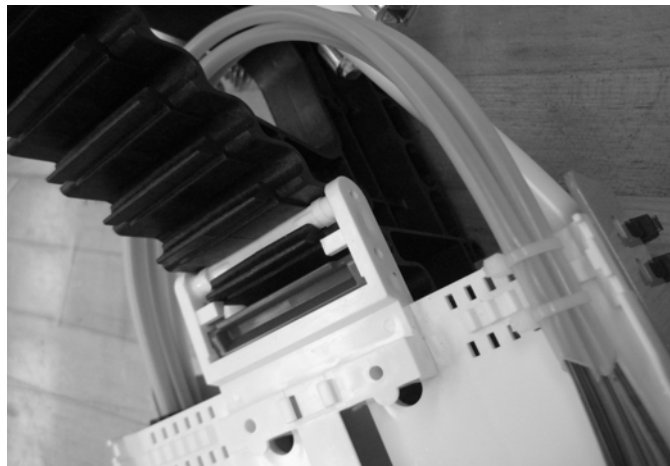
Figure 15 – Fasten transport tubes to splice tray.
