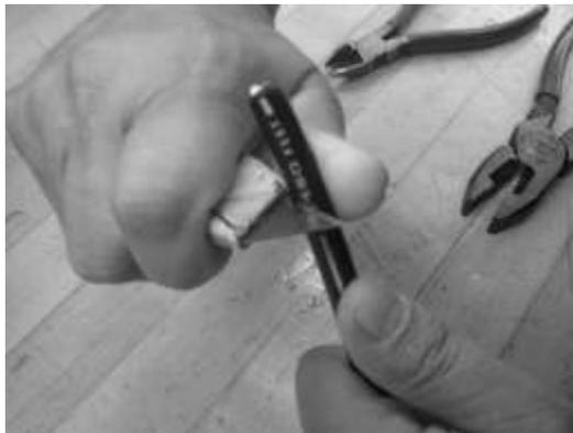
**Figure 1 – Ring cut the cable.**
