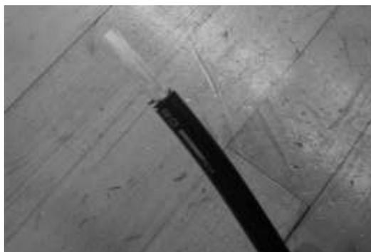
**Figure 2 – Remove the 3" length of outer jacket and armor.**
