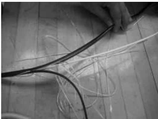
**Figure 4 – Separate the cable jacket into two sections.**
