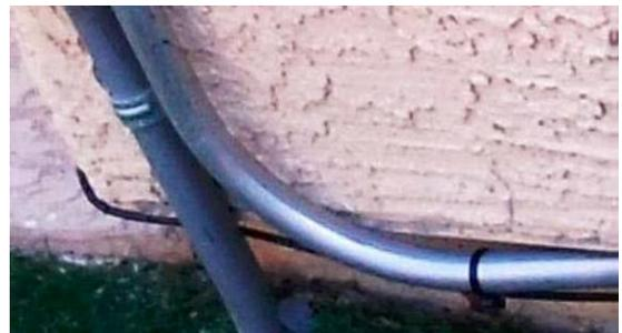
5.7 Installing EZ-Bend cable through a conduit into the attic of a home.
