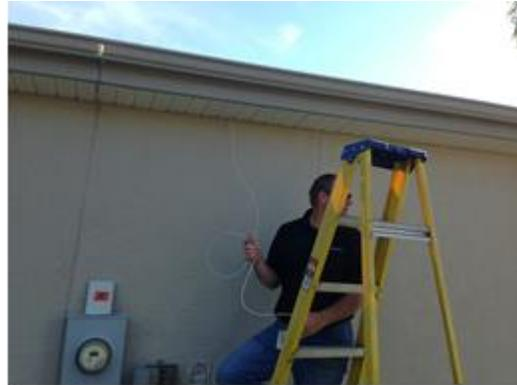
5.9 EZ Bend Cable can be fastened to masonry walls using shark tooth anchor clips<sup>3</sup> or similar fasteners.
