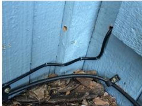
5.6 EZ-Bend cable fastened to an existing conduit using cable ties.
