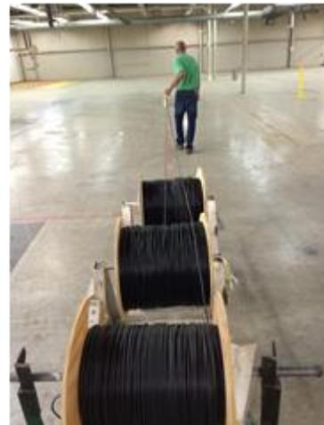
3.2 Inspect the cable reels for crossovers and/or slack coils which may get tangled during the pull. If slack coils are present, carefully pull the slack cable off the reel and neatly rewind. At the conclusion of the installation, staple the end of the cable to the reel flange to keep the cable tightly wound on the partial reels.
