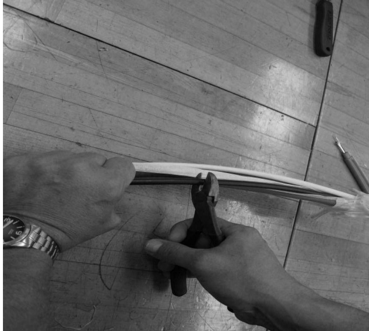
Figure 10 – Install strength member attachment bracket on cable.
