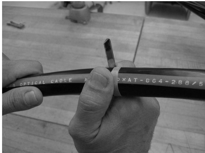
Figure 3 – Ring cut the outer cable jacket.
