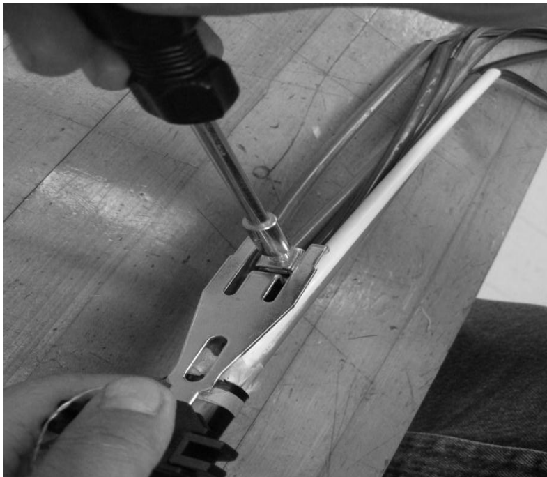
Figure 11 – Install cable attachment bracket.
