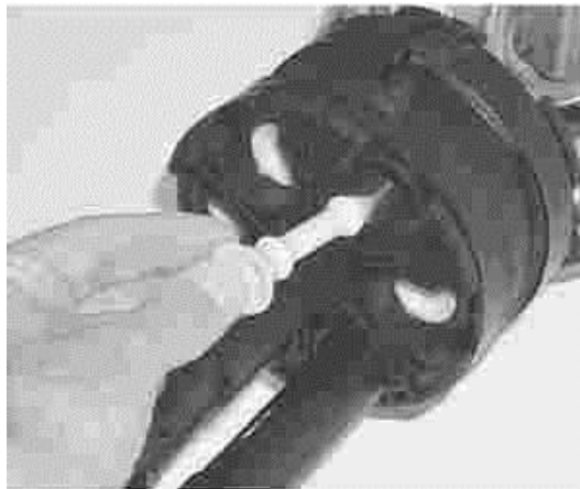
Figure 23 – Insert plugs into unused cable ports.
