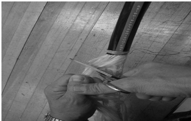
Figure 7 – Cut the rip cords and Kevlar.
