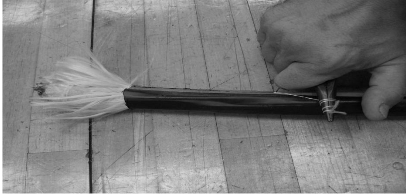
Figure 5 – Pull the ripcords through the outer jacket.
