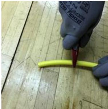
**3.4** Cut two parallel slits in the jacket between the outer ring cut and the end of the cable. The slits should be approximately 180° apart.
