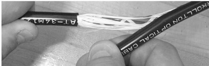
Figure 20 . Remove the 300mm section of outer sheath
