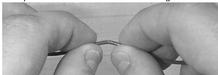
Figure 31 - Separate the buffer tube
