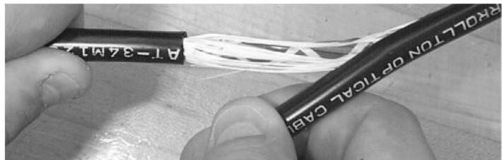
Figure 7 - Remove the outer sheath
