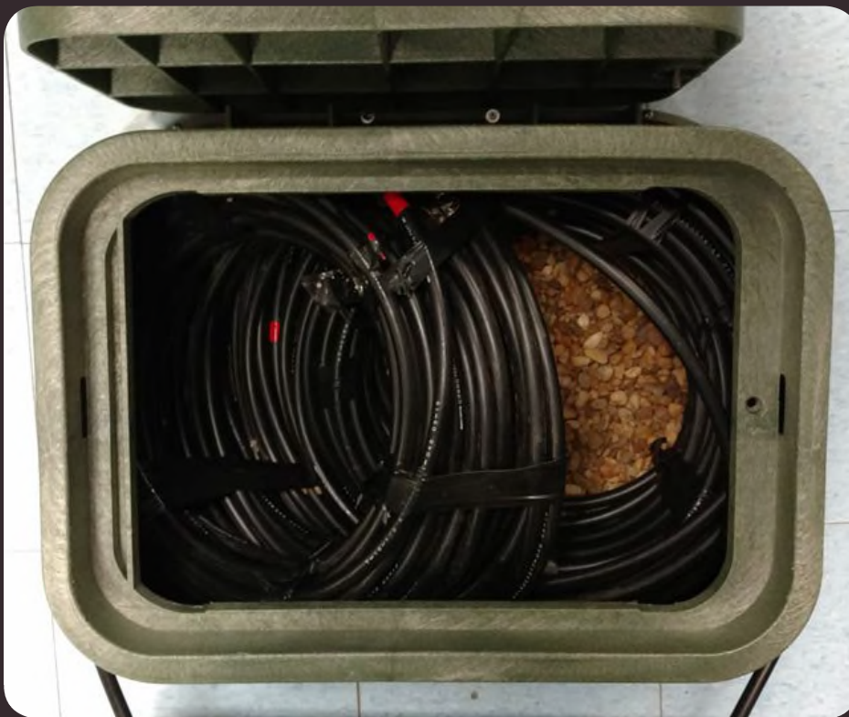
Figure 1. (a) Detail of the aggressive coiling of the loose tube cable in 12" diameter loops, (b) schematic of the optical loss testing performed in C and L-bands though the equivalent of a 97-km span.
